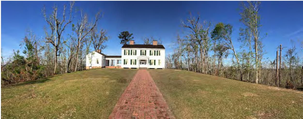
Figure 48. The Gregory House with canopy damage evident in adjacent slope forests.
