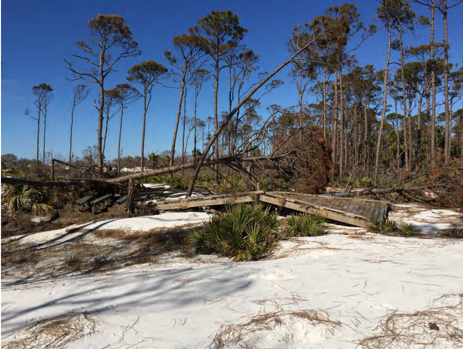
Figure 103. Sand deposition from nearby washed out dune and washed up portion of boardwalk in the Shady Pine campground.
