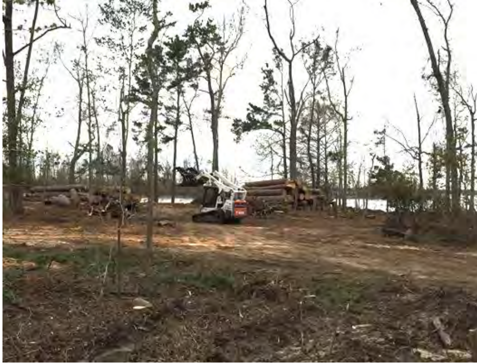
Figure 32. Campground during active cleanup of downed trees.
