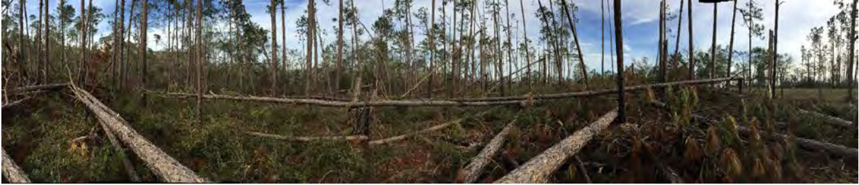
Figure 57. Older portion of the slash pine plantation with heavy damage in Zone TY-F.
