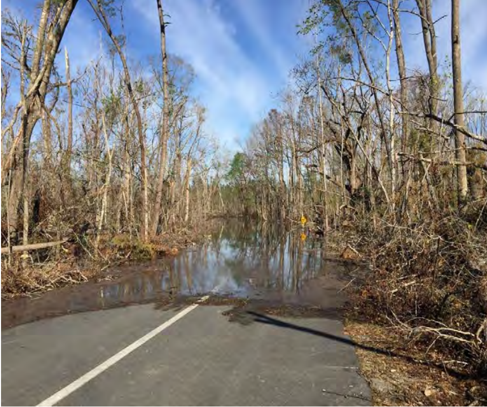
Figure 16. Flooding along Muddy Branch taken in the bottomland forest along the entrance drive. Flooding extended almost to the upland hardwood forest.
