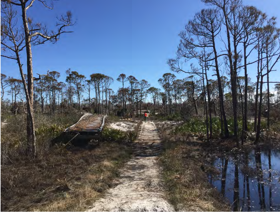
Figure 105. Boardwalk leading to beach access on the southern edge of the wilderness area.
